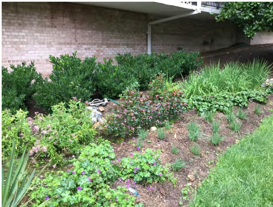
Figure III.G.7 The Waterford Condominium project: Fall of FY17 was filling in well after being installed in the Spring of FY16. This project demonstrated newer building techniques for rain gardens and is managing 2,700 SF of roof area.
