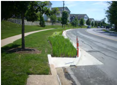
Green streets projects include (top to bottom) tree boxes, bioretention, and planted curb extensions.
