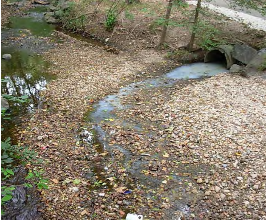
Outfall with milky discharge
